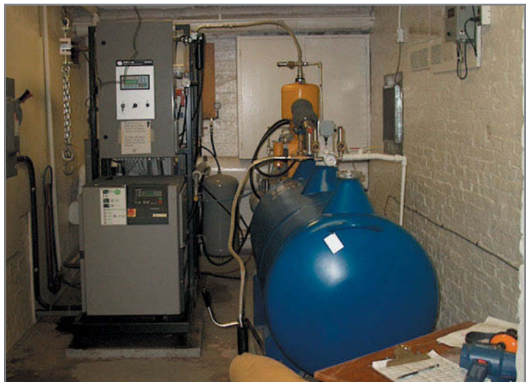
Photo 1 —This is the liquid nitrogen generator in its own small room. We don't dispense the liquid nitrogen directly from the blue tank, but rather transfer it to other dewars for actual dispensing outside of the room. The gray panel on the wall to the right is a unit I built that weighs these dewars in conjunction with a load cell and chain hoist visible at the left of the picture.
